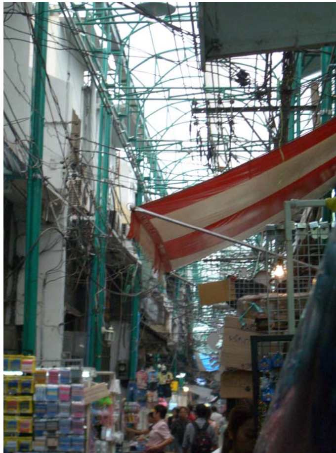
[alternative infrastructures: electrical wires in Bangkok]
